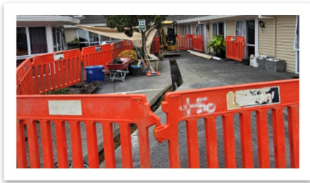
Drain improvement underway
