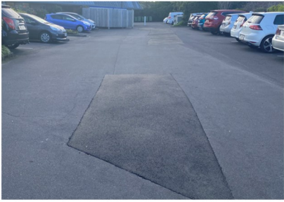
St Margarets parking area refurbishment
